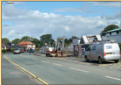
Extension to Caldew School
